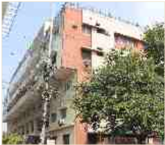
Atlas Apartments Road No.1, Banjara hills.
