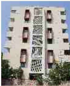
Mayfair Apartments Road No.2, Banjara hills.
